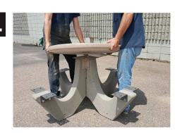
Mount table top and benches to installed brackets using (#10) neoprene pad and (#7) 3/8" x 1" hex flange bolts, four bolts per bench and top.
