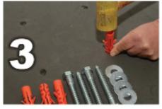
Use a rubber mallet or hammer to stuff mungo plugs into the drilled holes
