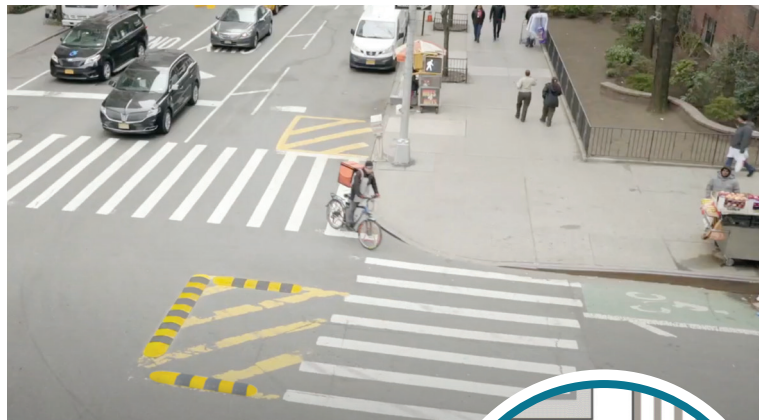
Bike Channelization Kit Installed where a one-way road meets a one-way road with a protected bike lane. This remedy was installed adjacent to existing bike islands.
