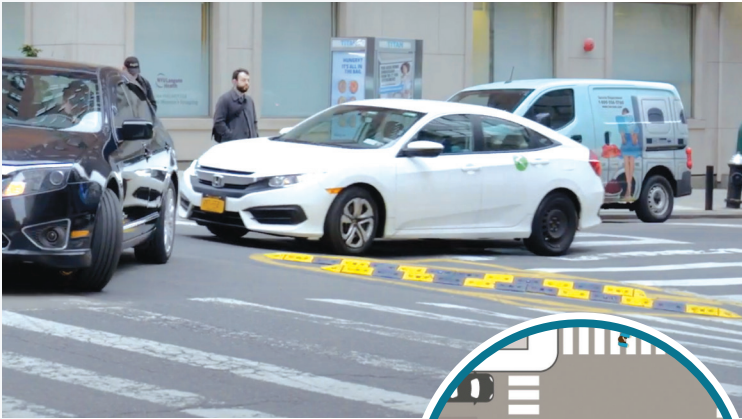
Complete Hardened Centerline Kit Installed where a one-way road meets a two-way road.
